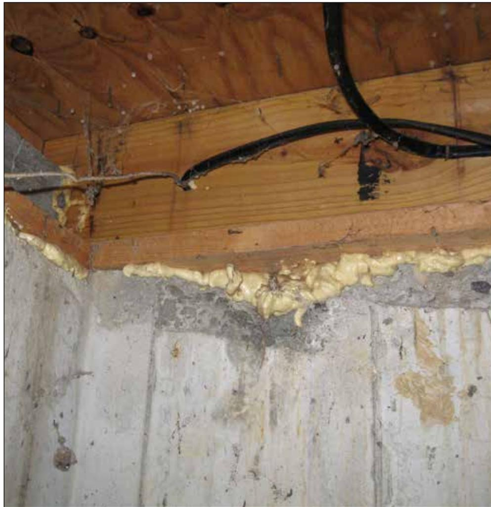
**ABOVE: Use expanding insulating foam to seal wiring holes and gaps where the sill plate rests on the foundation. BELOW LEFT: Place a foam draft sealer over the switch or outlet before replacing the faceplate.**
